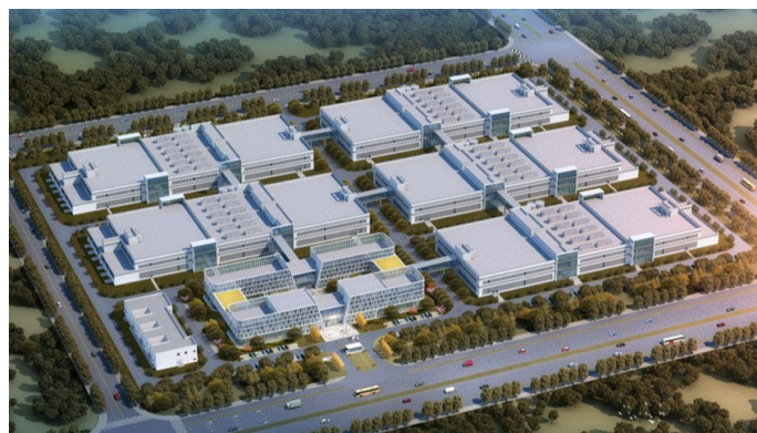
FIG. 1 Yucode Data Center in Ulanqab City, Inner Mongolia
